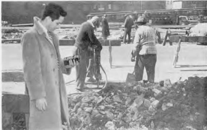
(Right) Figure 7. Sound-Survey Meter being used to measure noise level produced by pneumatic rock drills.
